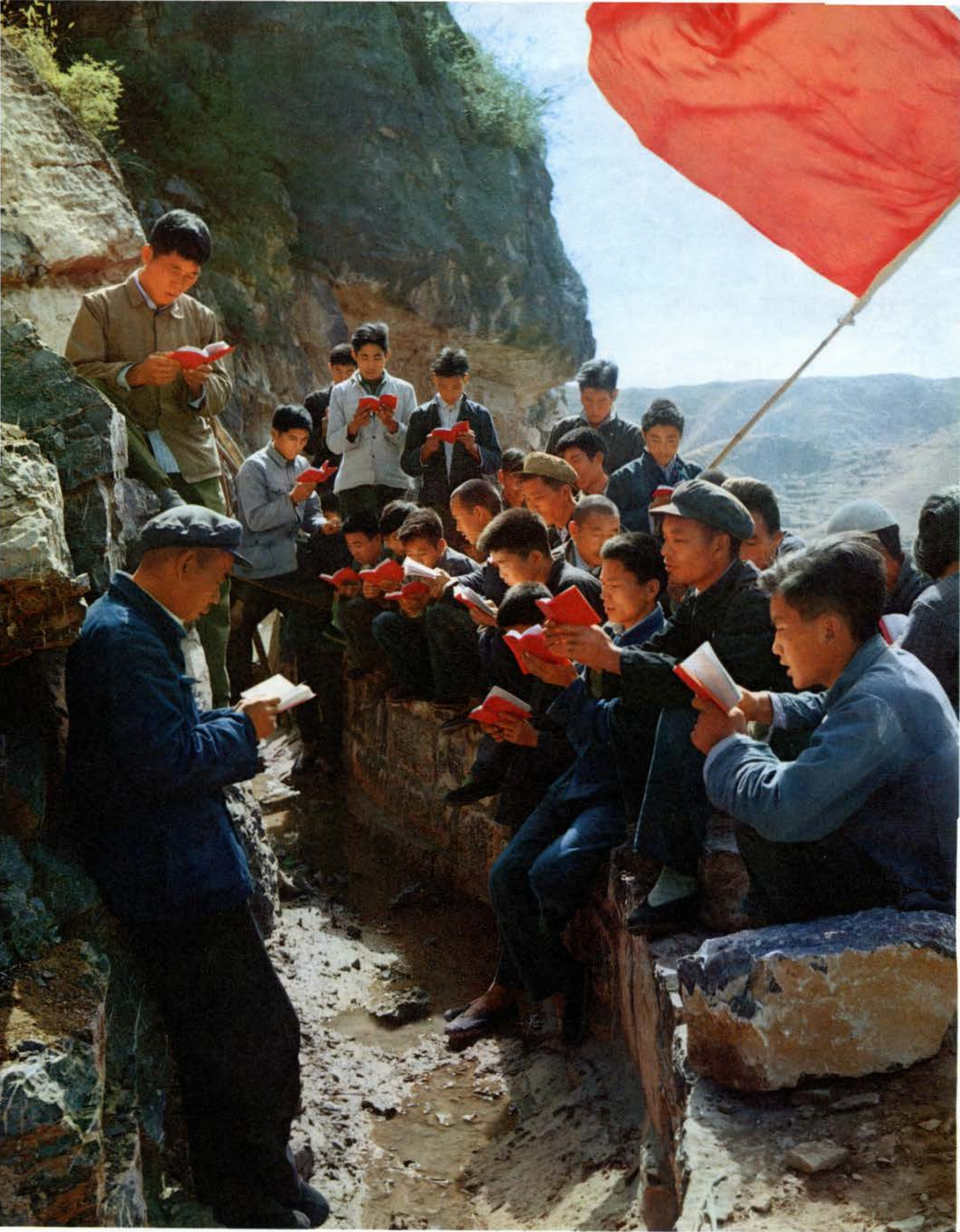
Creatively studying and applying Chairman Mao's works have become an everyday practice throughout Linhsien County. Builders of the canal are studying quotations from Chairman Mao at the construction site.
