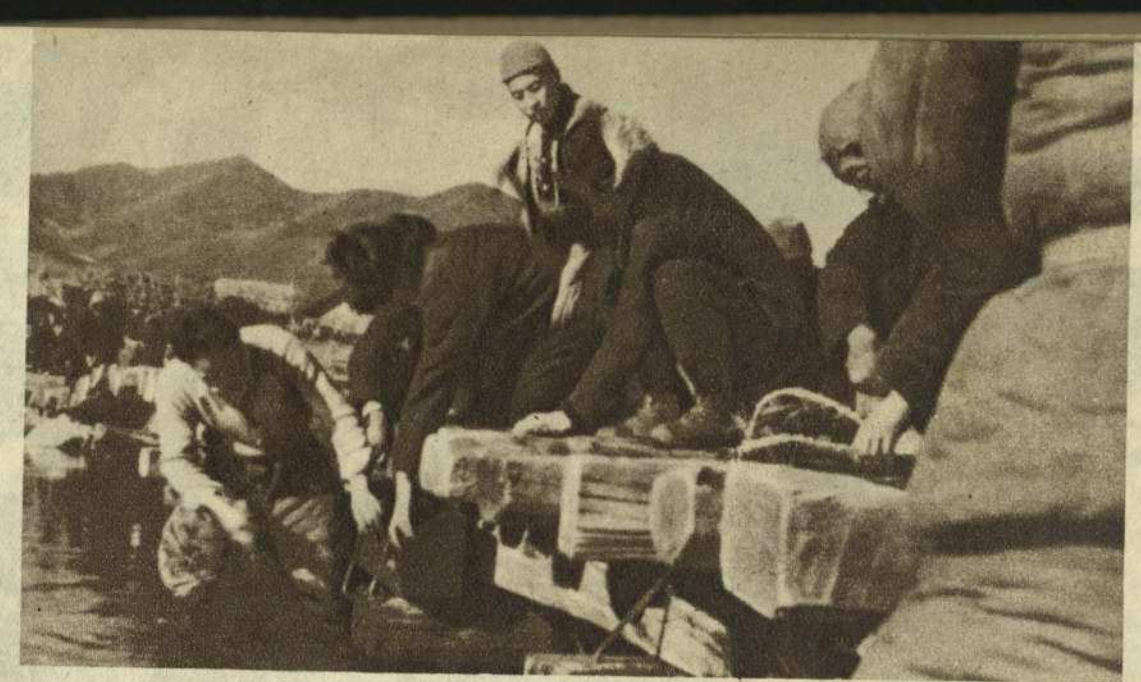
The volunteers assist Korean workers to repair a bombed bridge.
