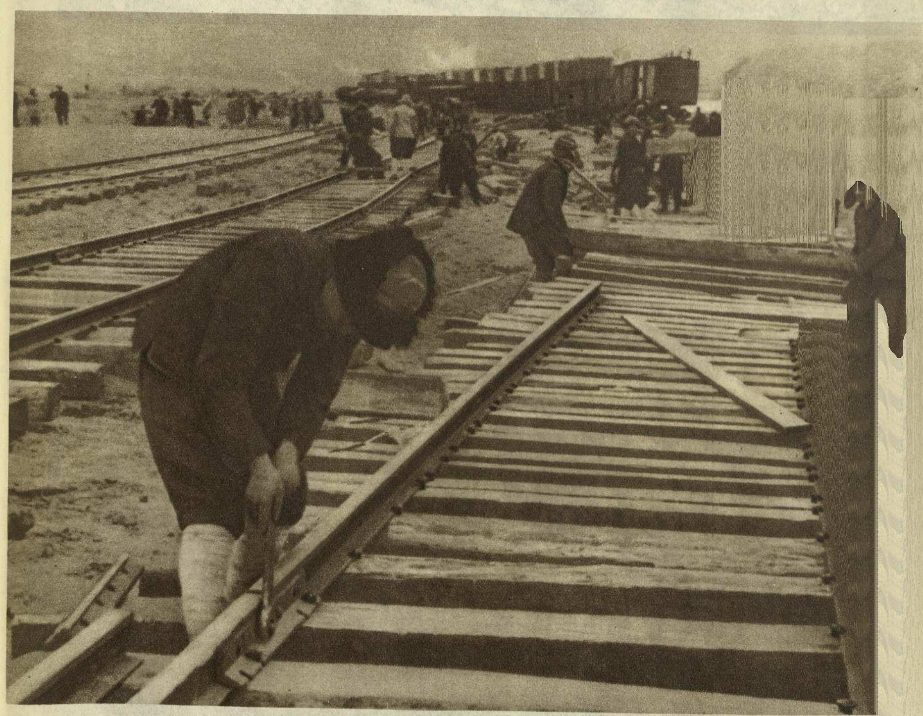
A bombed rail track is quickly repaired.
