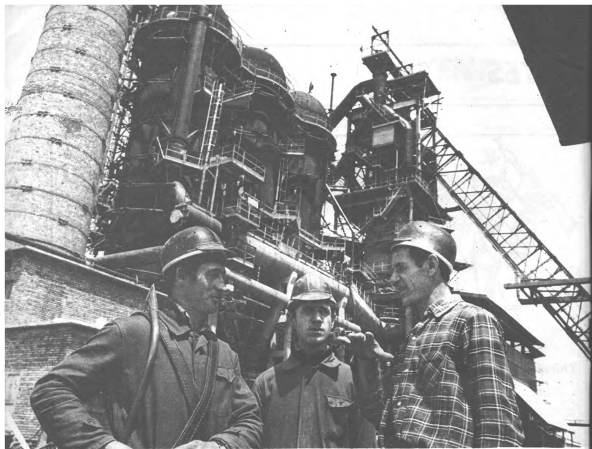
Builders of the furnace at the new metallurgical complex at Elbasan.
